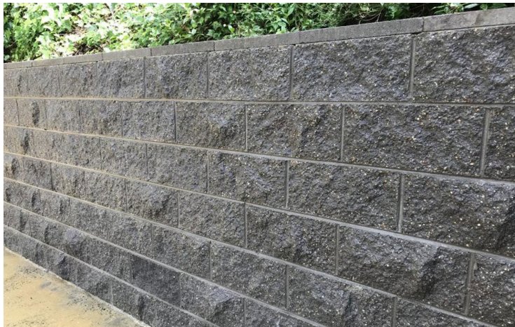
CMU Block Wall
