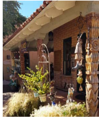
PAINTED WOOD EAVE
