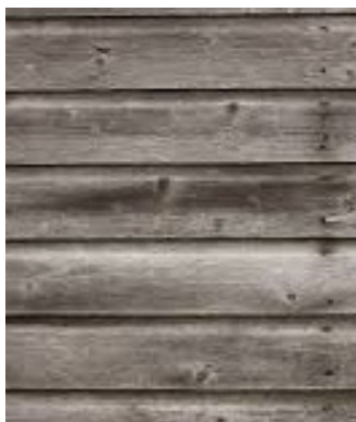
WEATHERED WOOD SIDING
