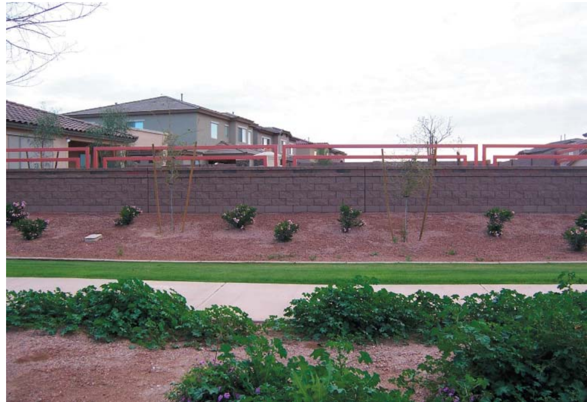
FIGURE 14: SIX FOOT THEME WALL ON BERM
