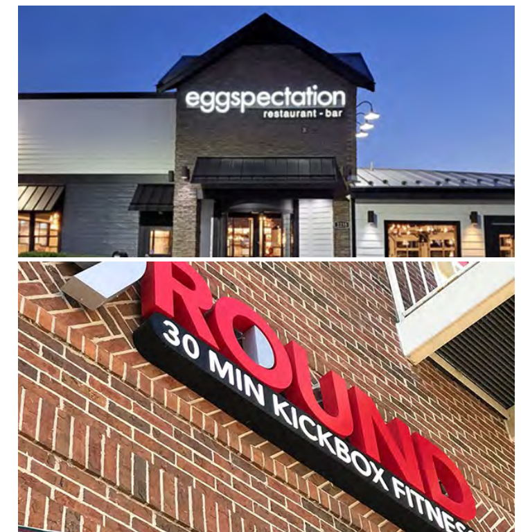
EXAMPLES: CHANNEL LETTERS WITH PUSH THRU CABINET FOR SECONDARY COPY
