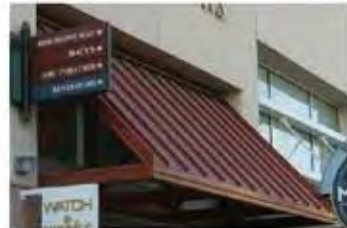
8 METAL AWNING IMAGE
