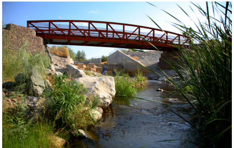
Trail Crossing with Bridge
