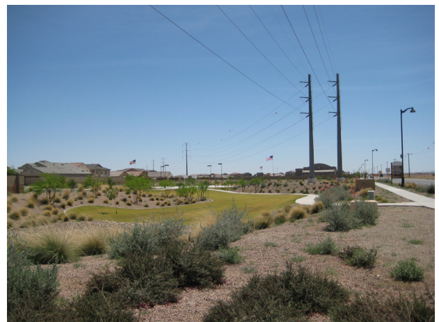
Powerline Corridor in the Eastern City of Maricopa Planning Area
