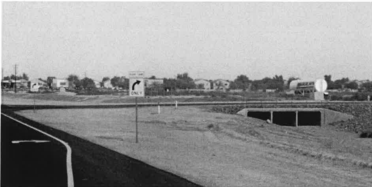
Example of box culvert at Copper Sky Park
