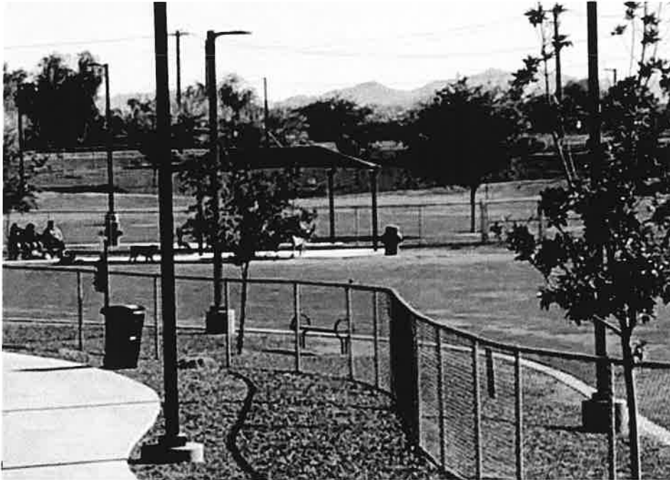
Existing Pedestrian Site Lighting at Copper Sky Park
